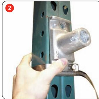
Wrap the hose clamp around the post and fit it into the groove on the mount.
